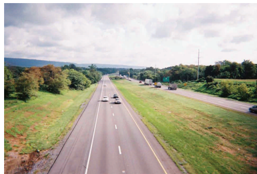
I-81 at Rich Valley Road
