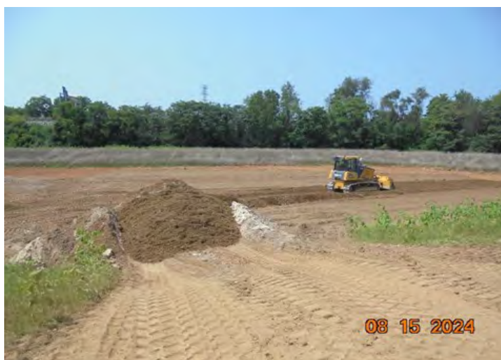
Amended soils (mix of topsoil and sand) being installed in an infiltration SCM.
