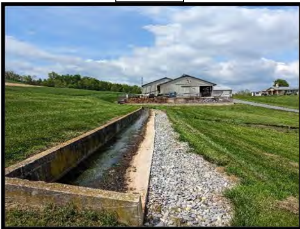
An outdated concrete level-lip spreader creates concentrated manure flow to a stream.
