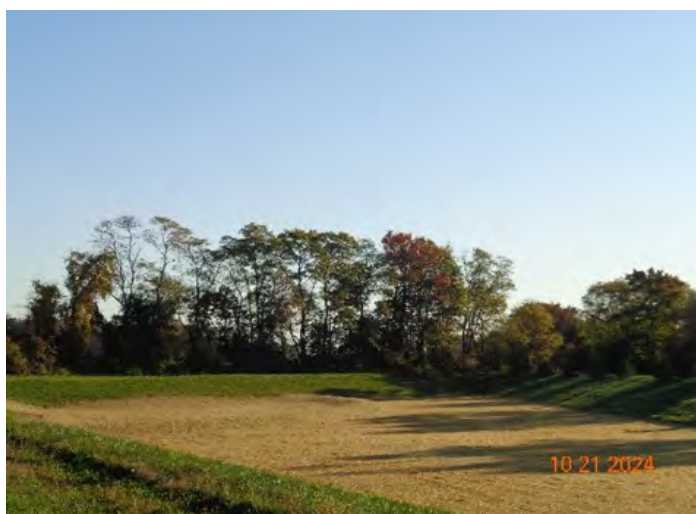
Infiltration SCM after the amended soil is installed and the floor is seeded and straw mulched.
