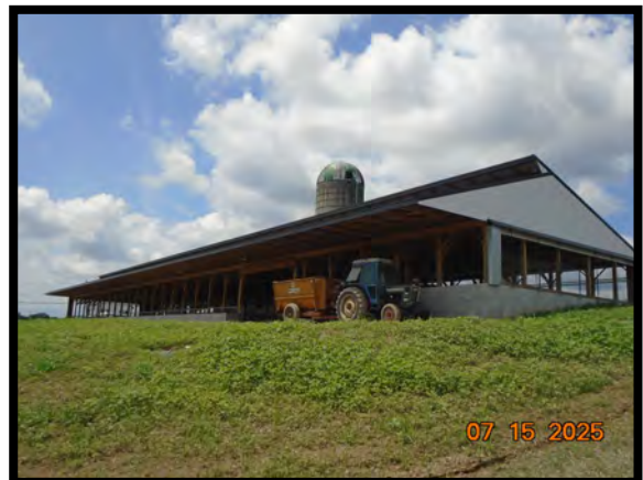
A roofed animal heavy use area was installed through the ACAP program to contain nutrients and keep the manure and cattle dry.
