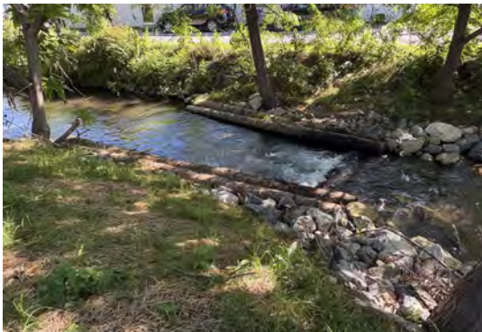
Cross vane installed in Middle Spring Creek
