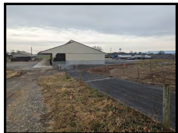
A cattle walkway with diversion belts was installed through the CEG program to improve the walking surface, divert rainwater, and discourage loafing to get cattle out to pasture.
