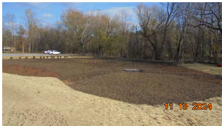
Picture of a rain garden planted with plugs acting as an infiltration stormwater control measure (SCM) at Willow Mill Park along the Conodoguinet Creek in Silver Spring Township. The rain garden will infiltrate runoff from impervious surfaces, which will reduce the volume and improve the water quality of the runoff prior to entering the creek.
