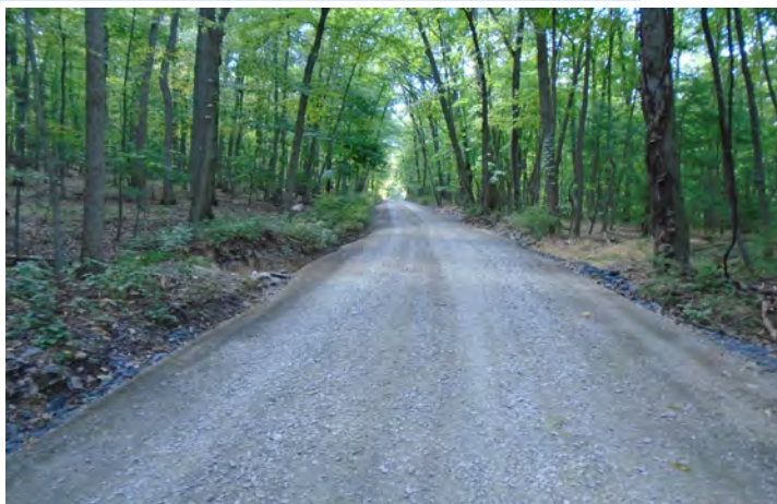
Ridge Road after implementing drainage improvements, shale fill, and topped with 2A stone.
