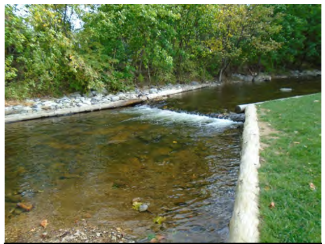
Previous project on the same stretch of Mountain Creek involving the installation of mud sills to prevent further erosion of the stream bank
