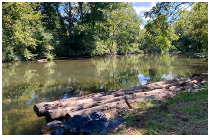
Log vane deflectors along the Yellow Breeches at the Woodcreek Development
