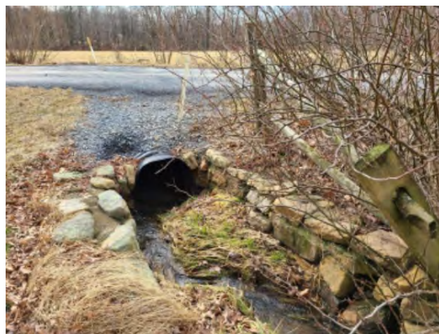
30 inch cross pipe on Pipeline Road Lower Mifflin Township
