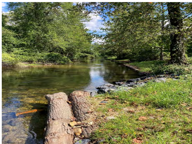
Log vane deflectors along the Yellow Breeches at Barnitz Church
