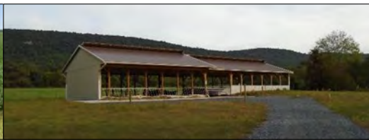
Roofed Heavy Use Area with Manure Stacking Pad
