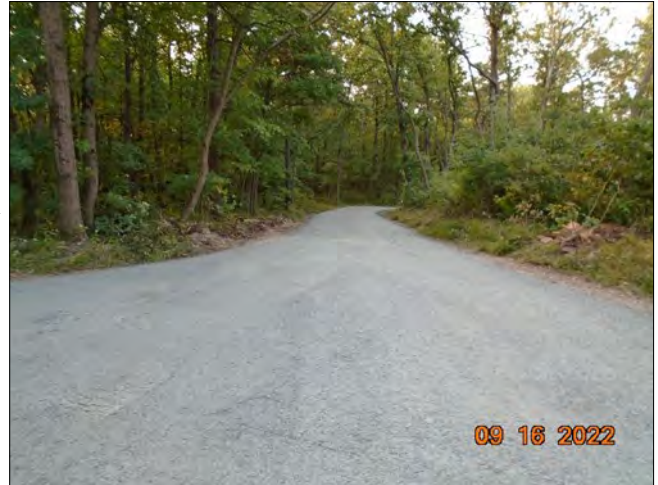
Above: Cold Springs Road (South Side) with completed Driving Surface Aggregate
