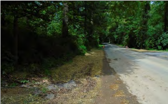
Left: Subsurface drainage ditch with topsoil surface
