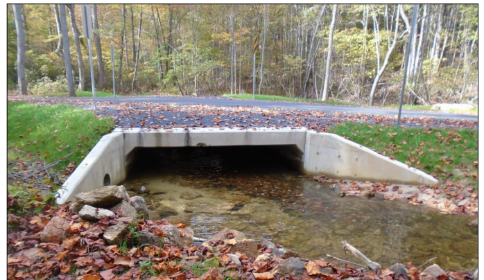
Penn Township, Beetem Hollow Road (Low Volume Road) Outlet of the stream crossing. The new culvert will reduce flooding and will allow for stream flow.
