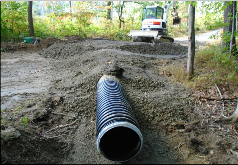
New shallow cross pipe installed with grade break to add additional road drainage.
