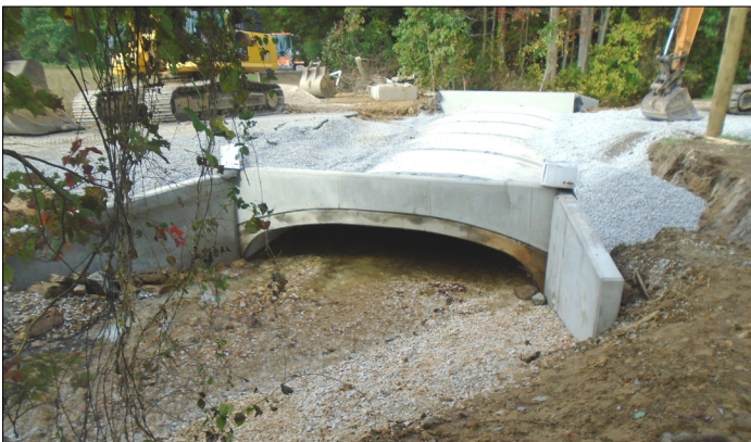
South Newton Township, Furnace Hollow Road (Low Volume Road) Inlet of the stream crossing. New culvert allows the stream to be connected through the structure and will prevent flooding.
