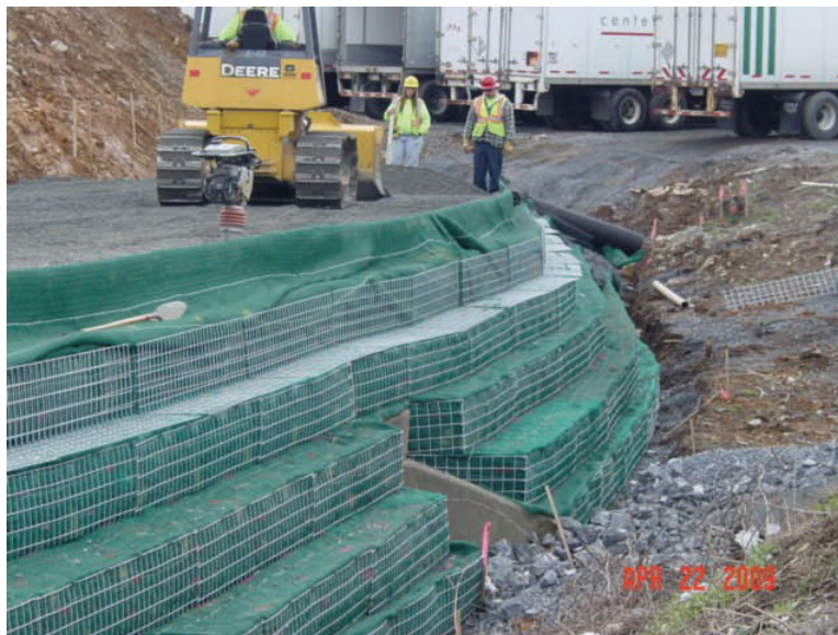
Geosynthetic Reinforced Stabilized Slope along ramp to U.S. Route 15.
