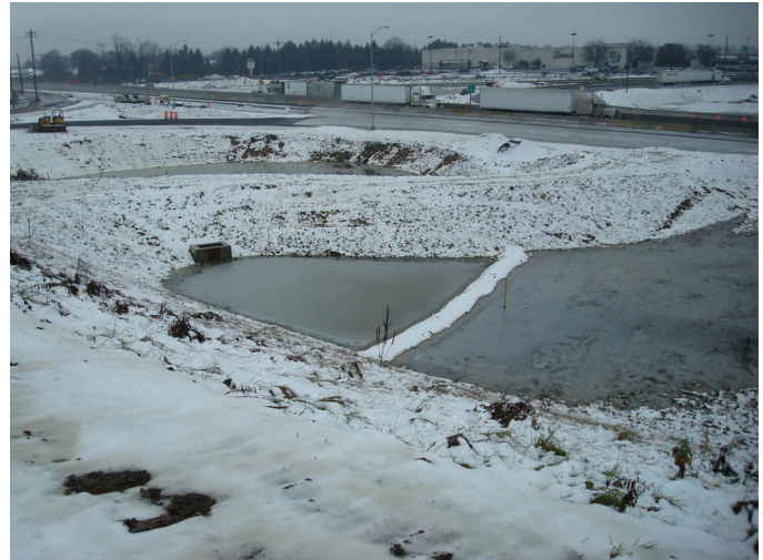
Sediment basins for Route 15 / 581 project.
