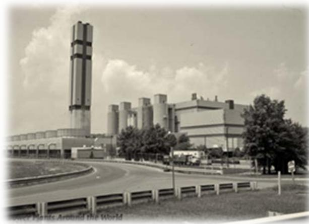
In RDF facilities, municipal waste is processed prior to burning. Essentially the combustible materials like paper, plastic, food and yard waste are mechanically
